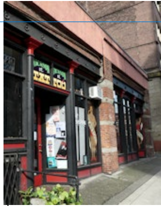
Figure xxx. Some buildings feature cast iron elements.
