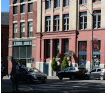
Figure xxx. An appropriate color palette for Pioneer Square: natural materials (brick and stone) complementary trim, and brighter colors reserved for accents and signs.
