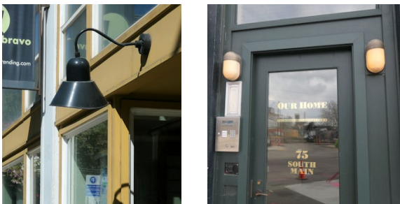
Figure xxx. Two examples of appropriate building mounted lighting. Note that it is particularly effective over building entrances.
